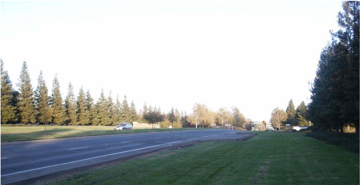
Figure 3.4-5. Wide planting beds on both shoulders and a center median bed (which is not continuous over the entire surveyed section) on Sunset Blvd. near Atherton. The extra wide shoulder areas are designed to accommodate future lane expansion. Coast redwoods on the left are on private property just beyond the City-maintained shoulder plantings. Most trees in this area are London plane and coast redwoods.
