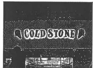
FLX FACED CHANNEL THROUGH FACE AND HALO & EXPOSED NEON WITH ALUMINUM FACE OVERLAYS
