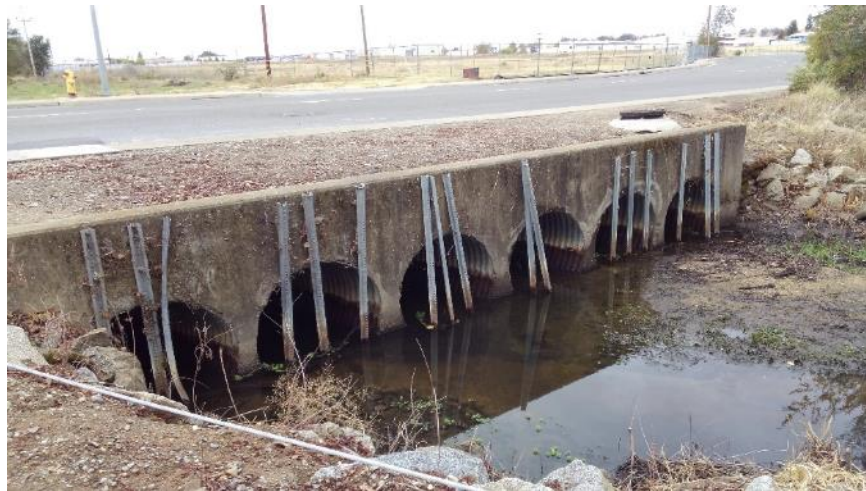
Description: Culverts located within the Brighton Preserve.
