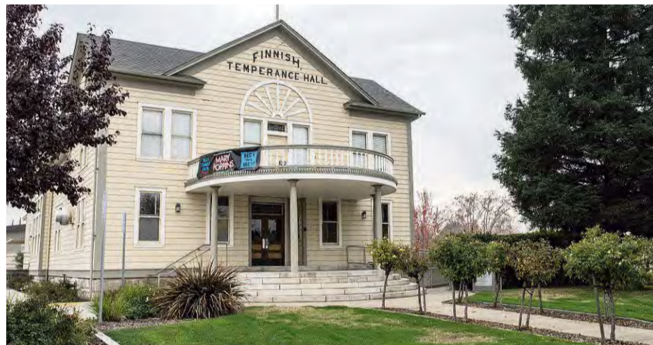
Finnish Temperance Hall is home to the Rocklin Community Theatre, which produces at least six shows a year.
